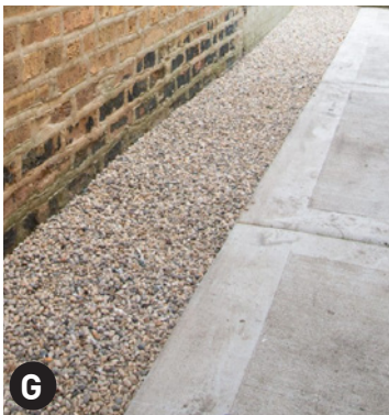
Maintenance Strip around building
